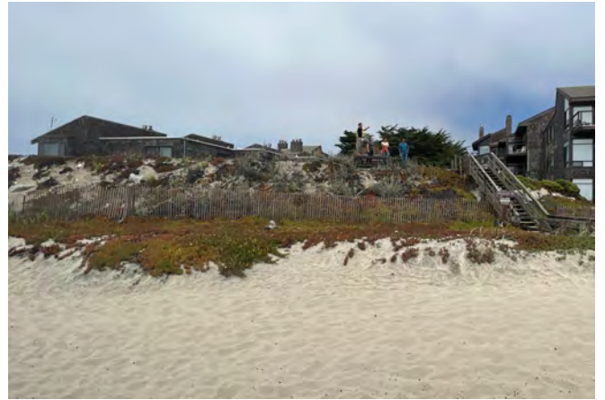
Photo 78: Pelican Drive - Complex B & C
