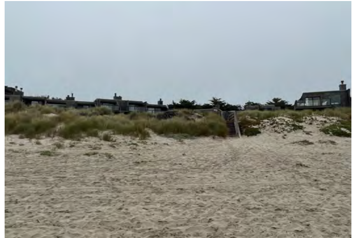
Photo 2: Units 8 - 14 Cypress Lane
