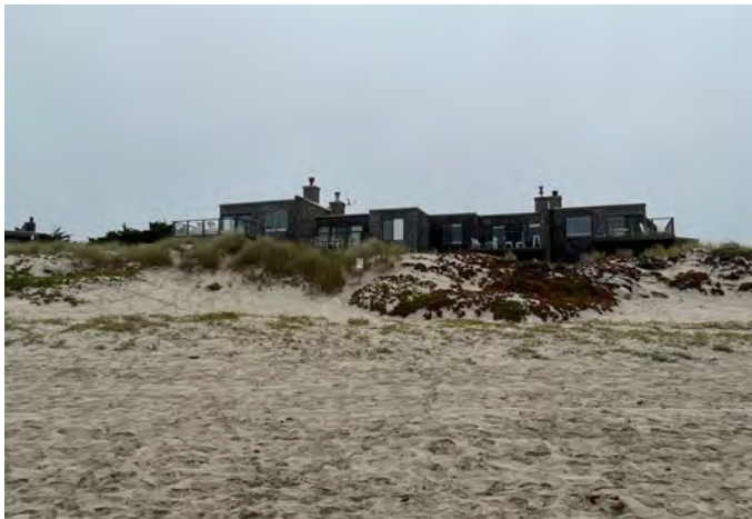
Photo 3: Units 14 - 17 Cypress Lane
