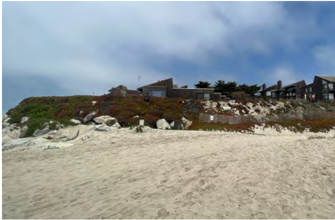
Photo 77.5: Pelican Drive - Complex B & C
