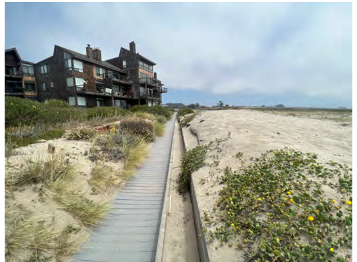
Photo 81: Sheetpile wall south of Pelican Drive - Complex C & D
