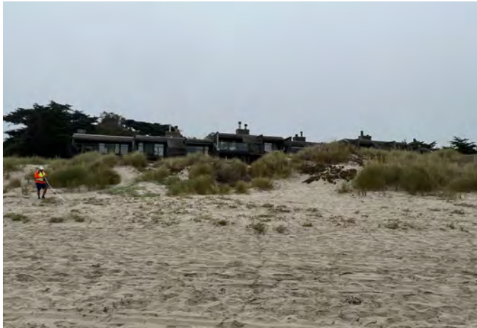
Photo 1: Units 1 - 10 Cypress Lane
