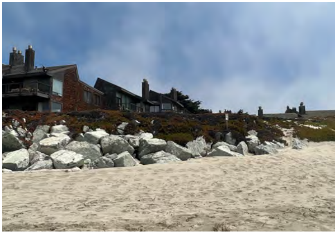
Photo 75: Pelican Drive - Complex A
