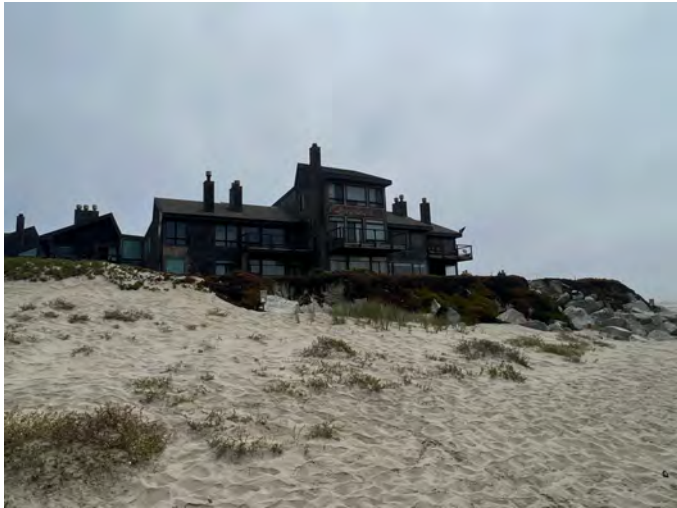
Photo 73: Pelican Drive - Complex A
