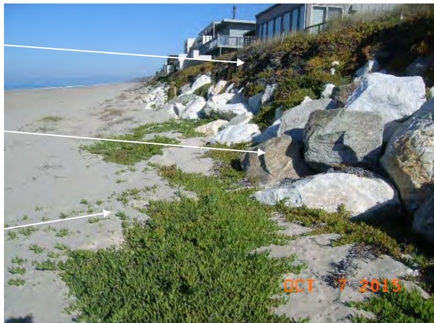
Figure 5. View of revetment repair project area, looking north from Lot 94, October 2015.
