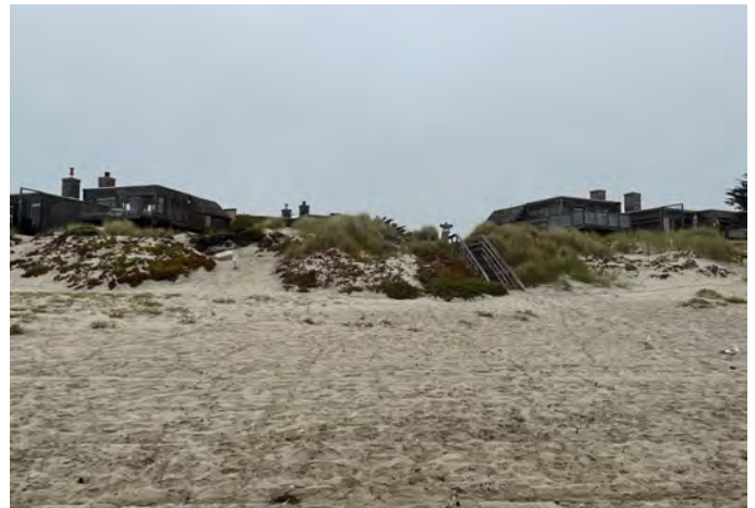
Photo 4: Units 17 - 20 Cypress Lane
