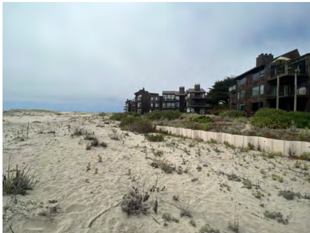
Photo 83.5: Sheetpile wall & dunes south of Pelican Drive - Complex D & E
