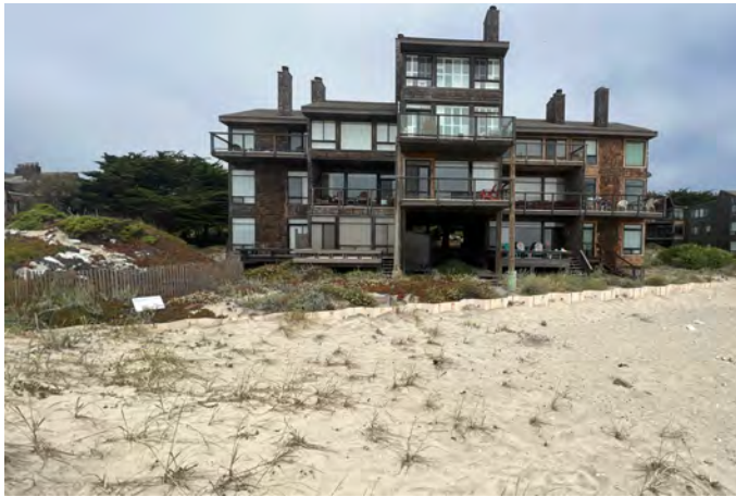
Photo 79: Pelican Drive - Complex C & Sheetpile Wall
