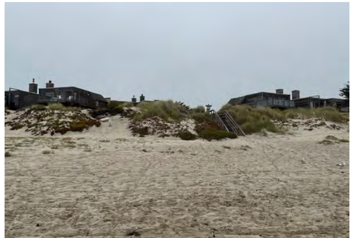
Photo 4: Units 17 - 20 Cypress Lane
