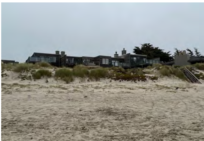
Photo 5: Units 20 - 23 Cypress Lane
