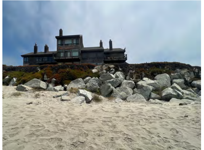
Photo 74: Pelican Drive - Complex A
