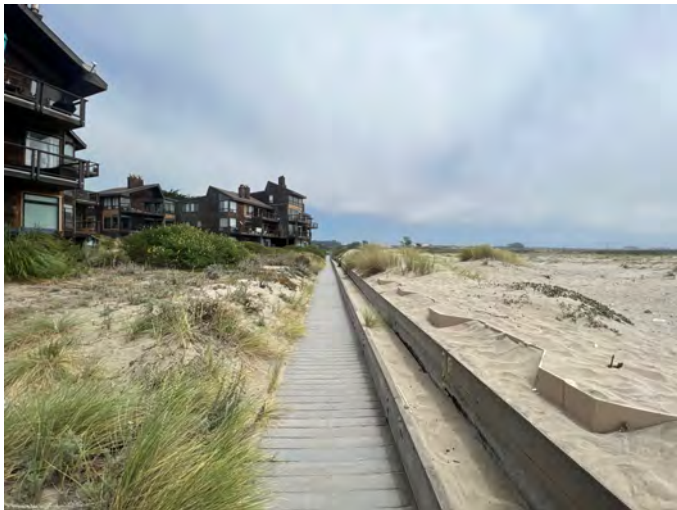
Photo 80.5: Sheetpile wall south of Pelican Drive - Complex C
