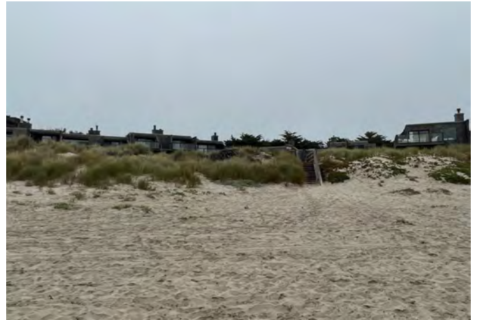
Photo 2: Units 8 - 14 Cypress Lane
