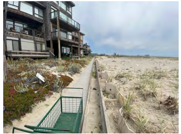
Photo 80: Sheetpile wall south of Pelican Drive - Complex C
